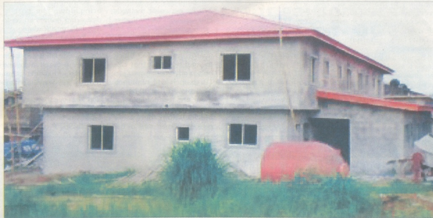
• A house being constructed by Cornerstone Construction Limited in Oregun, Lagos.
